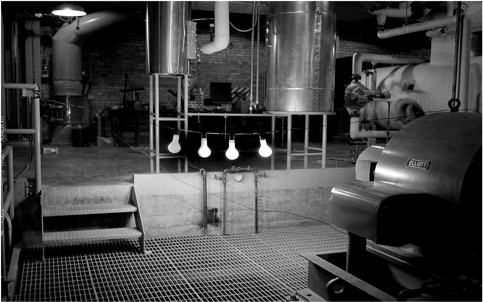
1951 - 65 Years ago - Experimental Breeder Reactor-I. By illuminating four light bulbs EBR-I became the world's first electricity-generating nuclear power plant
